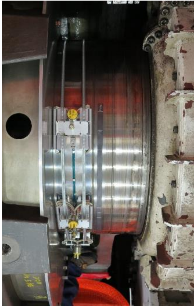
Shaft installation process
